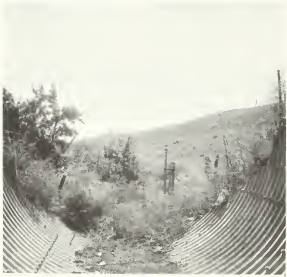
Looking East from EAST ENTRANCE
